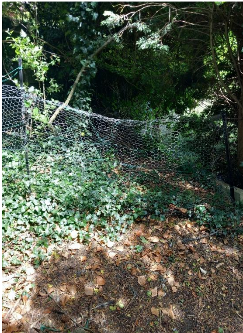
Photo 5 Only one section of fence remains upright
