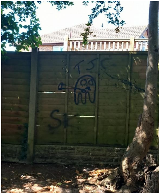
10 Graffiti within covered area.
