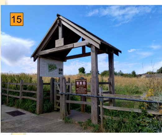
Bishop's Palace, entered through the gate displaying its history. Information boards record details of historic value.
