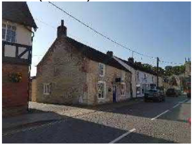
Figure 37 1 Church Street (Grade II).
