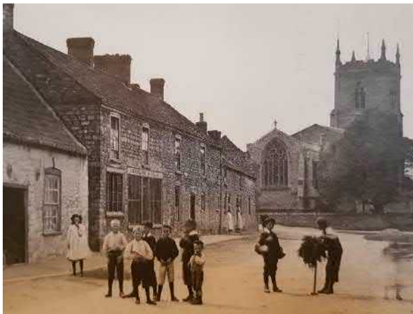
Figure 12 c.1904 image looking west along Church Street towards to the Church of All Saints. 69
