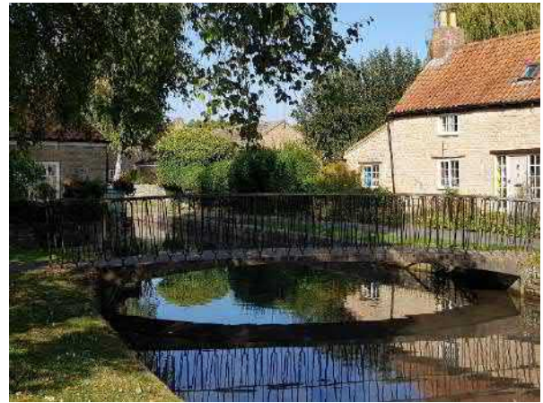
Figure 68 Concrete bridge with metal handrails across the beck on the High Street.
