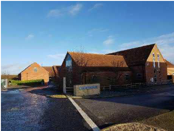
Figure 80 Example of commercial units in the business park on the north side of Deepdale Lane.
