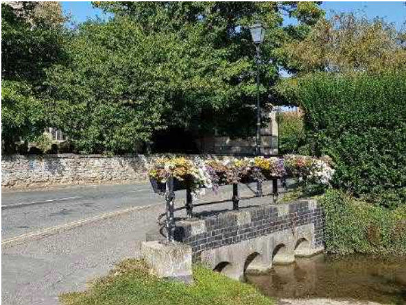
Figure 64 Jubilee Bridge with cast iron railings, flower planters and cast iron street lamp.
