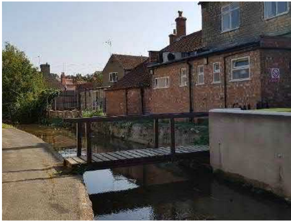
Figure 67 Timber modern bridge across the beck at the rear of the White Hart Inn.
