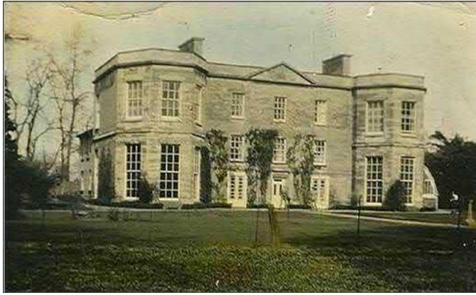
Figure 121 Nettleham Hall pre-1937, when it was left ruined by a fire. 83
