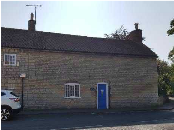
Figure 46 Coursed limestone of an asymmetrical facade on Church Lane.
