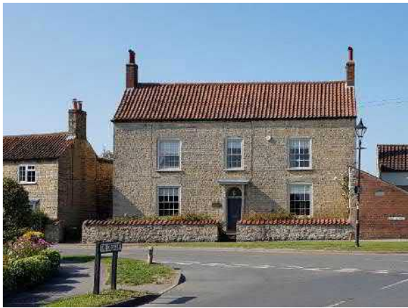
Figure 50 Limestone and pantile gabled roof of the former vicarage on East Street.
