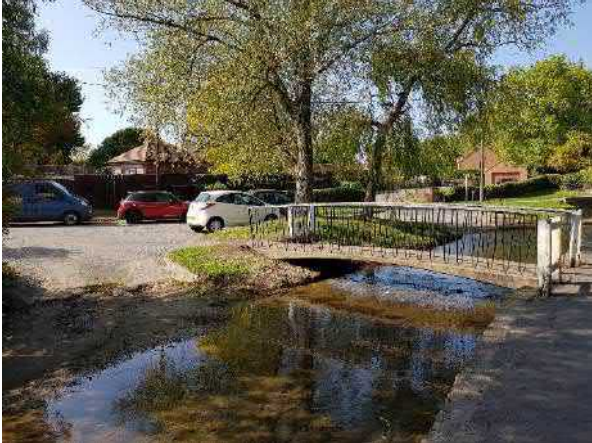
Figure 57 View looking southwest across the beck at the ford on Watermill Lane.
