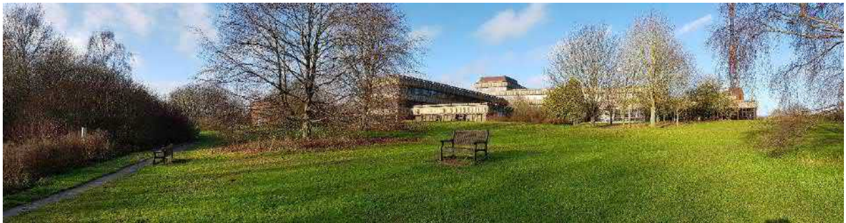
Figure 90 Police Headquarters panoramic view from the grassed area and public footpath on the south side of the complex.
