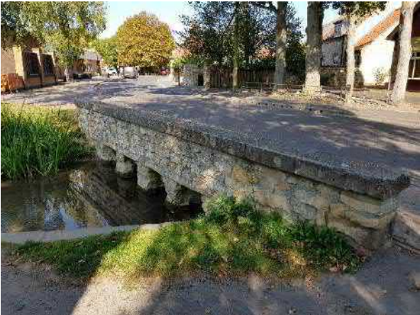
Figure 63 Road bridge at the north end of Vicarage Lane.
