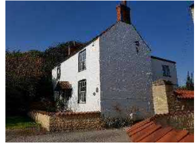
Figure 36 10 Church Street (Grade II).
