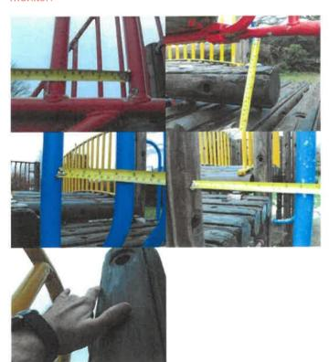
Opening on barrier greater than 500mm wide without a guard rail in place – *low risk* – monitor.
