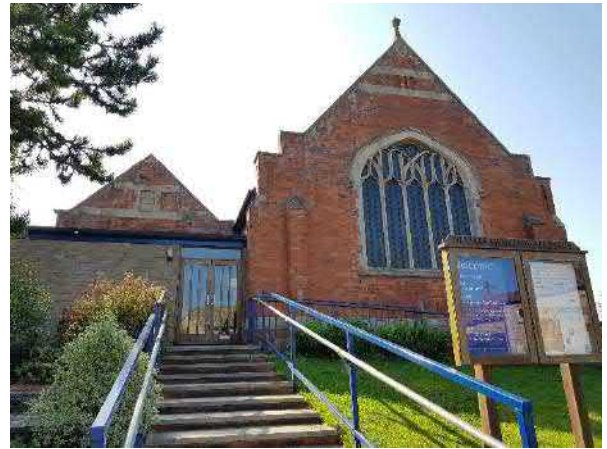
Figure 53 Red brick and stone dressing of the Methodist Church on High Street with a modern unsympathetic addition on the northeast corner.
