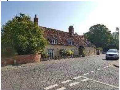
Figure 40 Beck House (Grade II) - Grade II listed Barn and stable range to rear of property. Believed to date from the 16 th century and oldest surviving building after the church.
