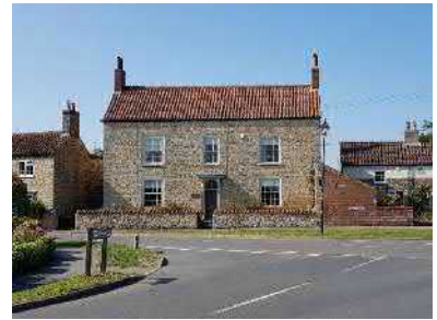
Figure 42 The Old Vicarage (Grade II).
