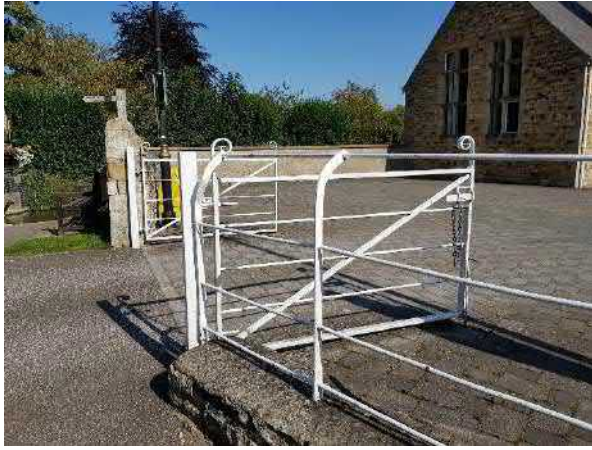
Figure 65 Wrought iron railings on low stone walls at the Old School at the south end of Church Lane.
