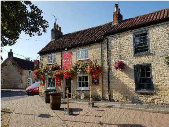
Figure 47 Limestone facades of the Plough Inn and neighbouring dwelling on the west side of the green.
