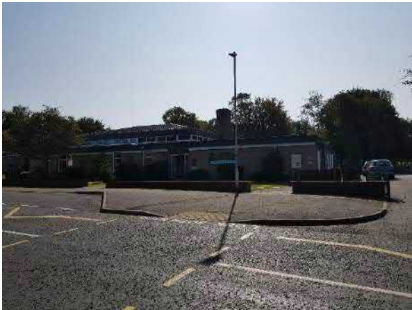
Figure 81 Nettleham Church of England Aided Junior School on the south side of the High Street.
