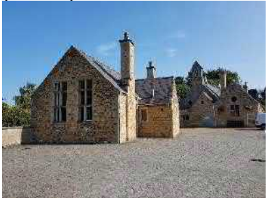
Figure 34 Old School and School House (Grade II).
