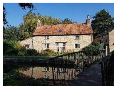
Figure 30 5 Becksides (Grade II).
