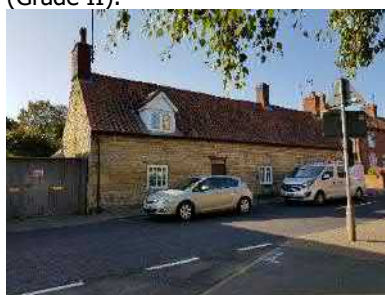
Figure 29 19 High Street (Grade II).
