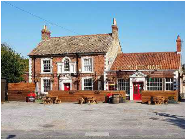
Figure 54 18 th century red brick with painted ashlar dressings of the White Hart on the High Street.
