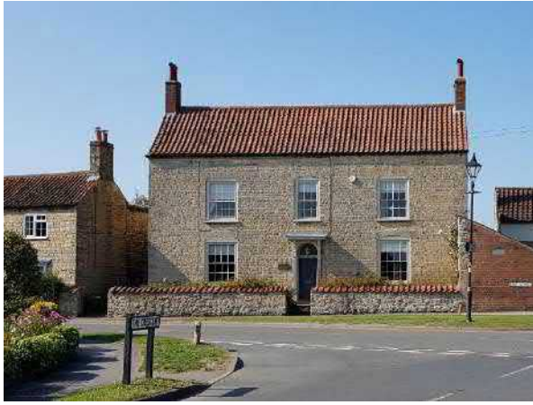
Figure 50 Limestone and pantile gabled roof of the former vicarage on East Street.
