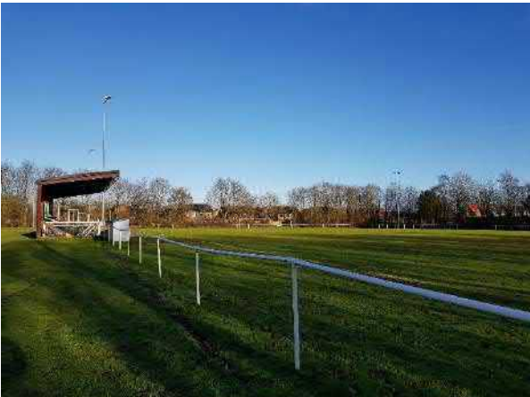
Figure 95 Part of the Mulsanne Park playing field on the east side, looking north.
