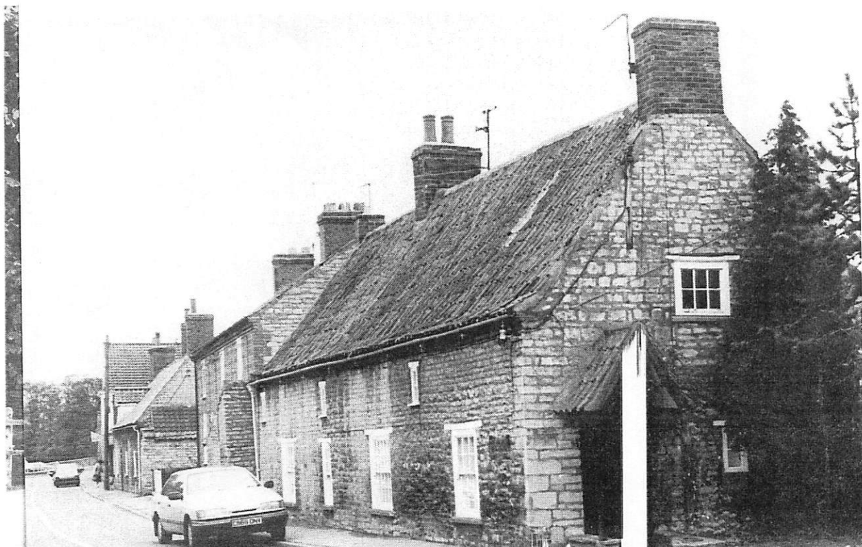
".... along the High Street .... (the buildings) .... are mainly stone built houses and cottages ...." para 15
